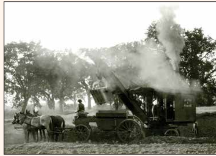
A steam shovel excavates rock and dirt and drops it in the wagon.
