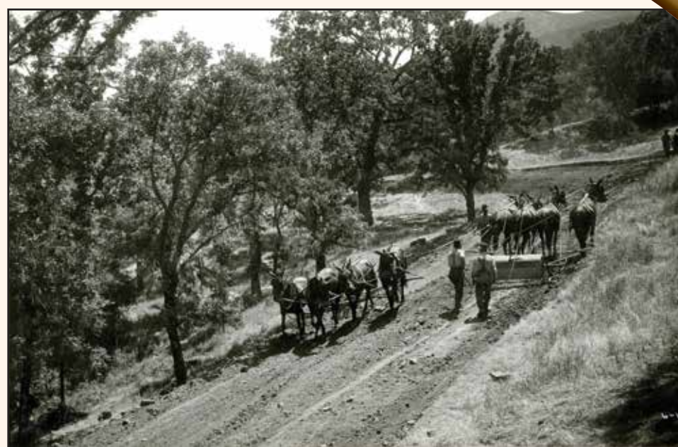
A Fresno scraper is used to flatten and level the ground. Here, the scraper gang gets a fresh mule team.
