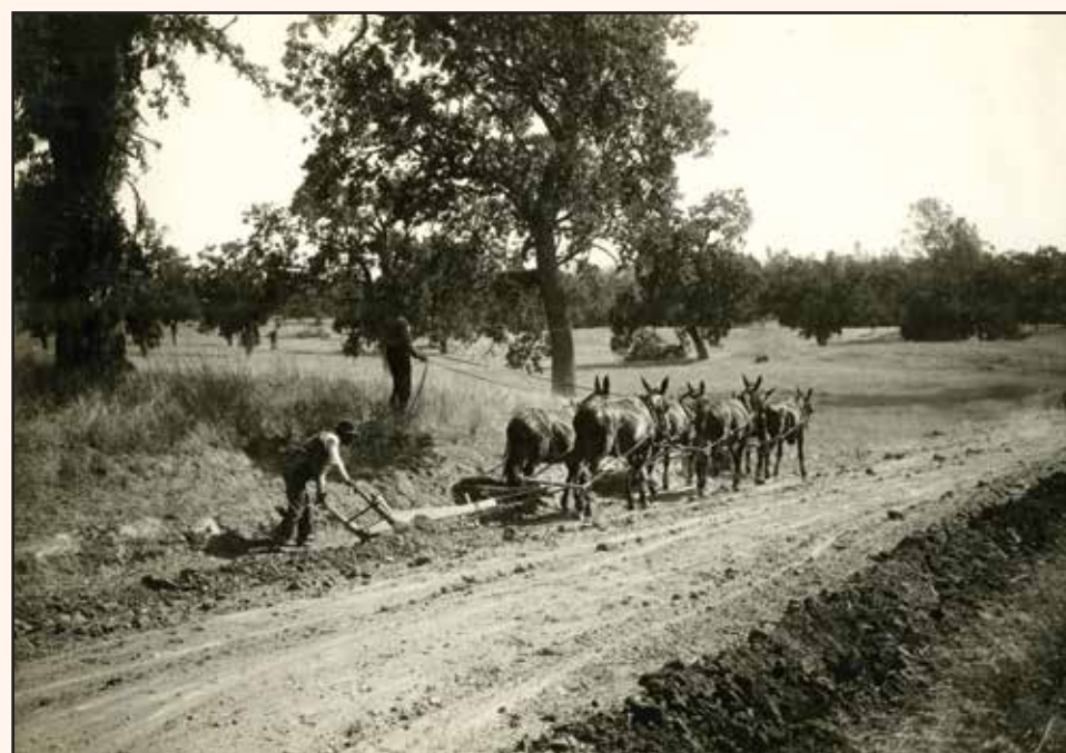
A grading blade is used to create drainage ditches and perform finishing touches to the road.
