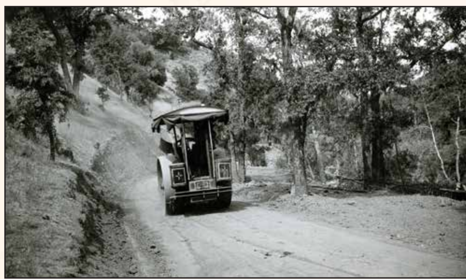
A roller smooths the surface.
